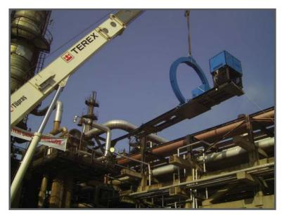
New "COBRA" line self-balancing fully electronic aerial extraction able to remove or reinstall bundle with or without your operator!
